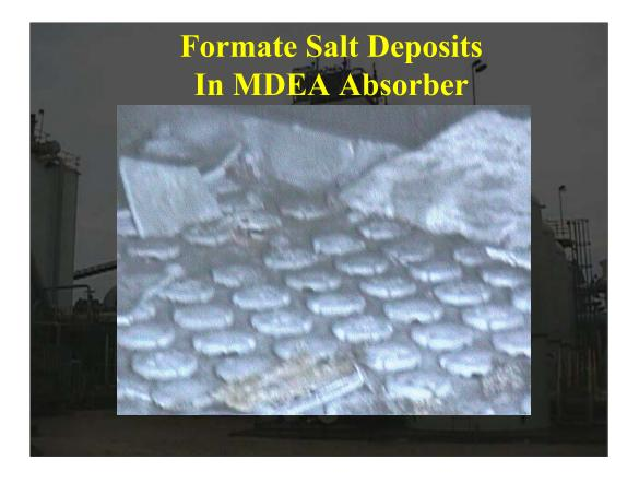
Heat stable salts from the reaction of formic acid produced by the COS hydrolysis catalyst with the acid gas removal solvent MDEA reached the saturation level in the circulating solvent. The salts deposited on the valve trays of the acid gas absorber shown here. Some of the salty mist also carried over from the absorber and plugged downstream equipment.
